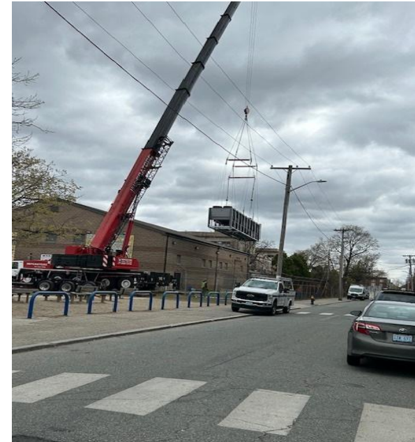
New Lima chiller being installed
