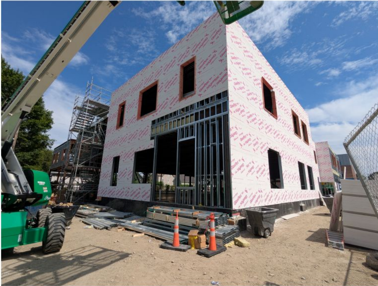
Exterior framing and sheathing underway
