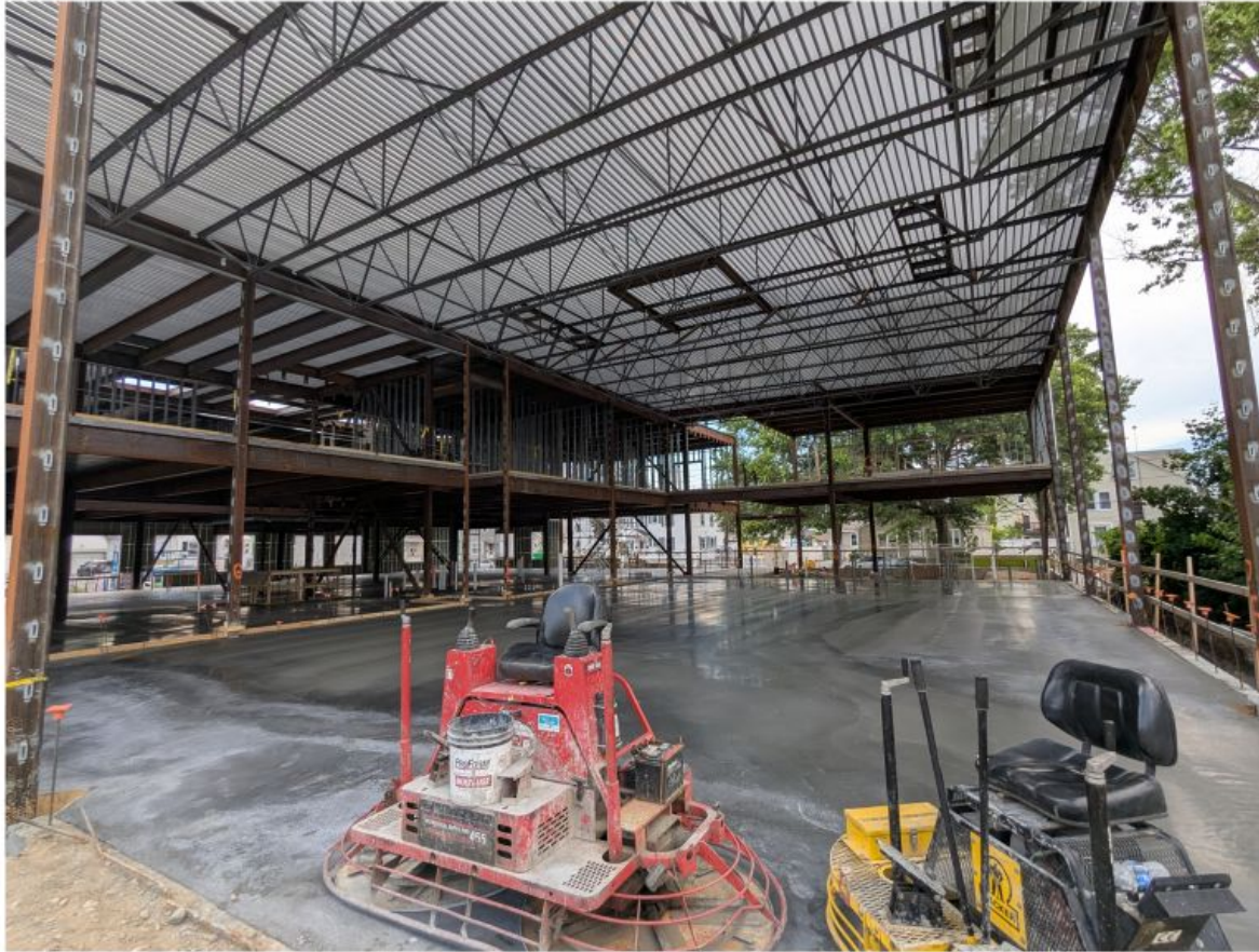
Slab on grade poured – view of Gym/Cafeteria
